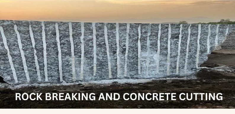
RAPID-CRACK (EXPANSIVE MORTAR) IS SAFE, EASY TO USE AND COST EFFECTIVE. IT DOES NOT NEED HEAVY EQUIPMENT, PERMITS AND SPECIAL CERTIFICATION.
